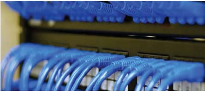
The structured cabling system in any given building is the catch-all term for the combination of smaller elements including the entrance facility where the building is connected to the outside world. Vertical distribution cabling connects multiple floors while horizontal cabling systems connecting various elements on a single floor, possibly through one or more telecom rooms. These rooms house switches, routers, power sources and other distribution equipment.
