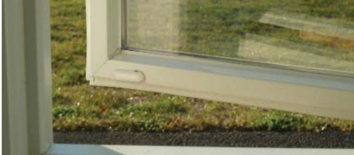
A typical magnetic switch has two halves, electrically wired to complete a circuit. One half of the pair is mounted on a stationary door or window frame as seen on the figure at the left. The other half of the magnetic switch is mounted to the movable portion of the window or door.
